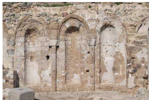
Figure 3. Northern wall of the crypt.
