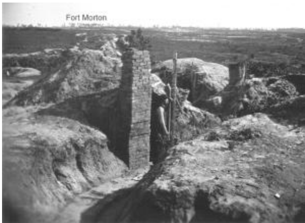
Figure 4. A photograph of the Petersburg battlefield that was taken shortly after both armies left the area. While the location of this photograph is not certain, it appears likely that Fort Morton appears here in the distance below the identifying text, and just below the horizon. An earthen parapet is seen there, along with several embrasures (openings for cannons). The person standing next to the brick chimney is probably a photographer's assistant.
