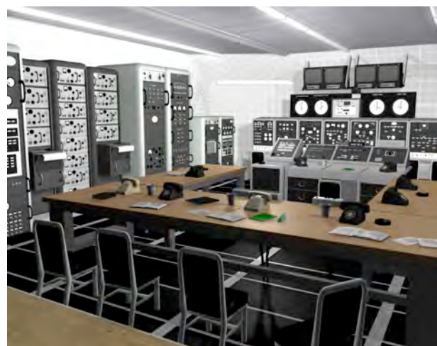
Figure 7. Interior Launch Complex 14 Blockhouse
